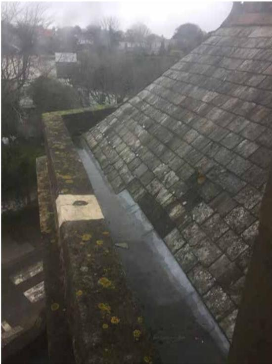
Loose, slipped and cracked slates to the roof have caused water ingress in the past, causing damage to roof timbers and ceiling/wall plasterwork. It is proposed to strip the existing roof slates, re-use as many as possible in re-tiling the roof and introduce breather membranes and insulation to the roof voids to improve the thermal efficiency of the building for the occupiers and users. Lead work will also be renewed to valley gutters and parapet walls.
