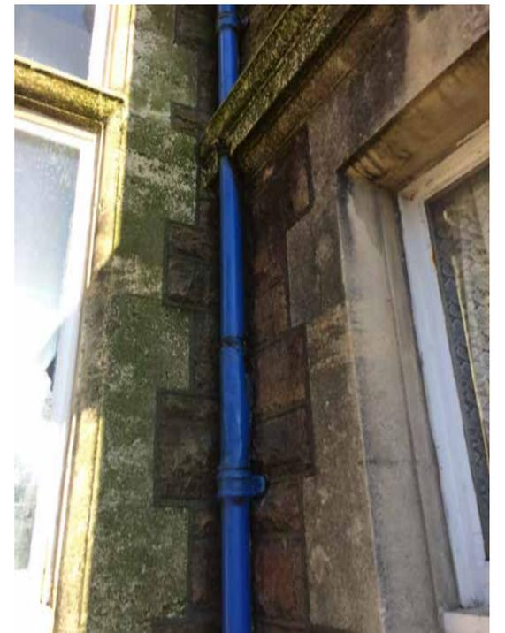
Blocked and damaged rainwater goods lead to water penetrating the building fabric and causing damage to the plasterwork and fittings internally. We propose to replace the existing rainwater goods with cast aluminium heritage range products and increase the sizes to allow for the future effects of climate change.
