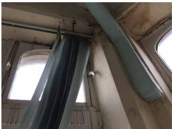
Although existing windows are in fairly sound condition, many require minor maintenance and redecoration. In certain areas of the building, it is proposed to install secondary glazing to improve the thermal efficiency of the building and reduce noise. In other areas, the use of thermal blinds will also assist with retaining heat within the building.
