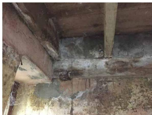
The existing tower roof timbers require replacement, together with the lead covering. Repairs to the roof will allow the reinstatement of the flag pole as in the Architect's original drawings for the building, allowing the Camborne Town Council flag to be prominently located.
