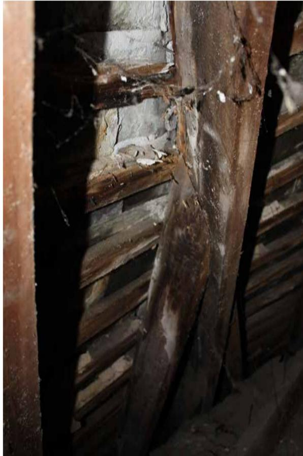
Damage caused to the roof timbers internally through slipped/cracked slates and water penetration will require localised timber repairs/replacements, with the roof space also being treated with a timber preservation solution.
