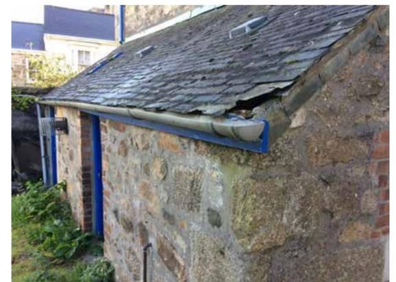
The existing boiler house is in need of repair, with the scantle slate roof failing. As the boiler is to be replaced and upgraded, the boiler house too will be repaired and re-roofed.
