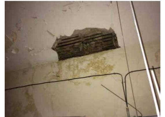
Damaged ceiling and wall plaster work as seen here, is caused by the lead trays to chimneys above failing and allowing water to penetrate the building over a long period of time. All damaged plaster work will be sensitively removed and replaced like-for-like and redecorated.
